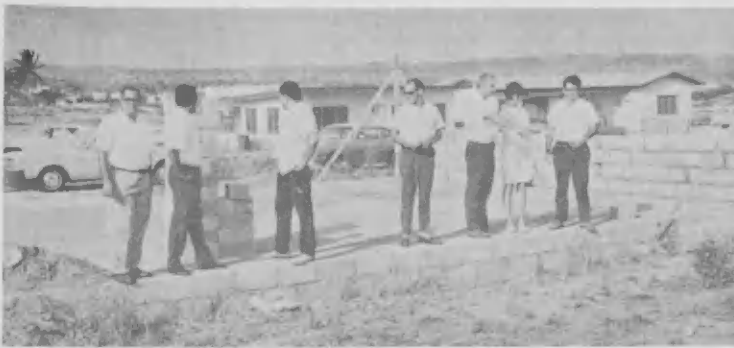
Board members and members of Aruba Amateur Radio Club (l to r in picture) J. H. Hassell, M. Angela, J. Geerlings, H. Schenkel, C. C. Lieffers, Mrs. Lieffers and J. Noguera inspect progress of construction on their clubhouse near Casa Cuna May 4.
